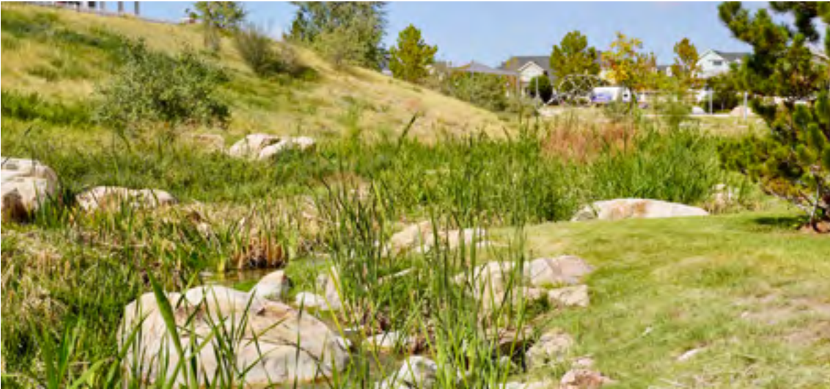
Grading and drainage Improvements are to focus on minimizing disruption of the site
