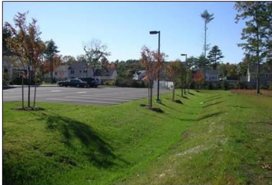
Figure 11: Vegetated Swales
