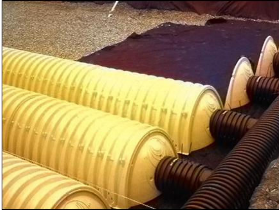
Figure 4: Underground Infiltration Gallery
