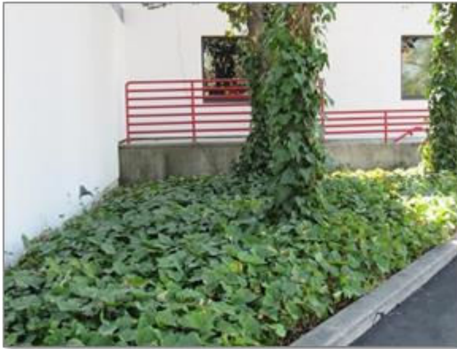
Figure 1: Downspout into Landscaped Area
