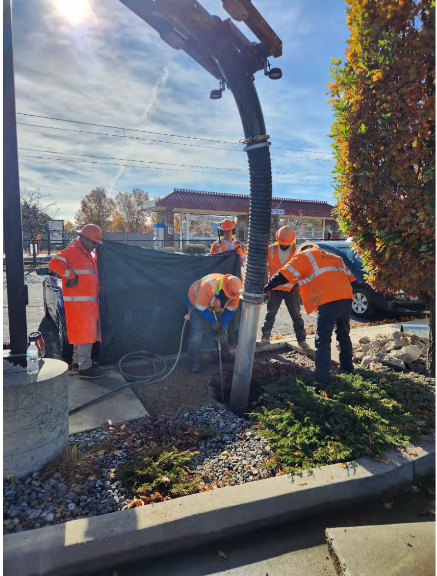
West Jordan Public Utilities crew using a hydro-excavator
